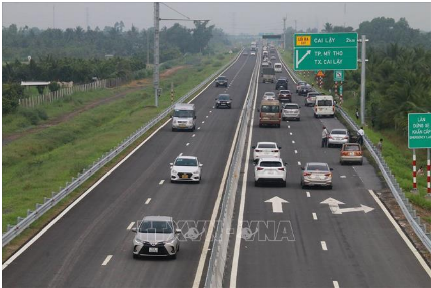
Ho Chi Minh City - Trung Luong - My Thuan Expressway (Phase 2)
