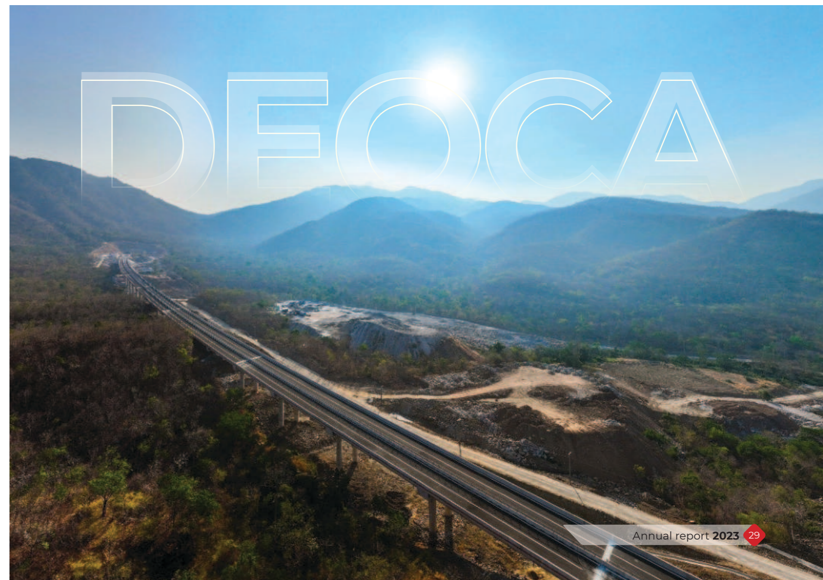
Cam Lam – Vinh Hao Expressway Project
