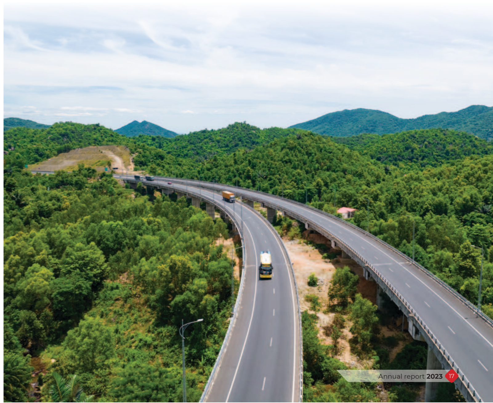
Deo Ca tunnel project
